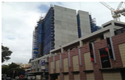
Burwood NSW 128 Units
